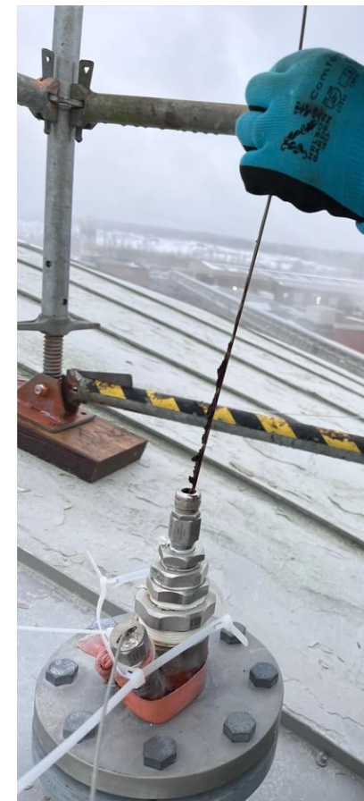
Installing the 10m fiberoptic temperature probe with 100 measurement points
